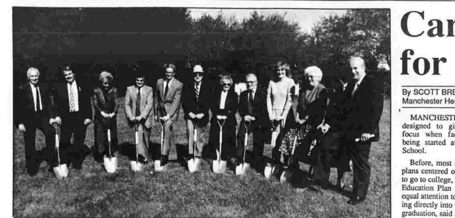
GROUND BREAKING — State and local officials joined members of the Housing Authority of Manchester Tuesday for the groundbreaking of a new elderly congregate housing complex in town.
